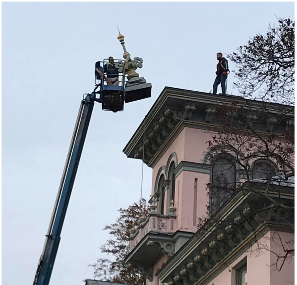
Right: Jon Pauldine stands atop the house museum while Dave Bock lowers the removed finial to the ground.
